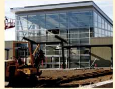
New Science Building under construction.
