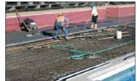
Workers pour and smooth concrete into the new pool decking.
