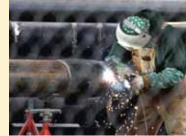
A new state-of-the-art Central Chiller Plant is scheduled to be completed in October 2007. A local firm, Bell Products, Inc., is working on the $7.2 million cooling plant. This green project includes a two-story building to house cooling towers and pumps. The facility will be used to create one million pounds of ice at night, while electricity rates are lowest, and then distribute chilled water to campus buildings for cooling during daytime hours. Daytime pumping will be solar powered thanks to the college's new photovoltaic field. Left, workers move one of the eight 10-ton chiller plant units into place as it floats on compressed-air jacks. Above, a welder seals seams on piping destined for the new chiller plant.
