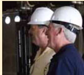
Napa Valley College Campus Planning & Construction Director Dan TerAvest, left, and Project Coordinator Pat Marrinan observe the delicate placement of one of the eight chiller units being installed in the new building.
